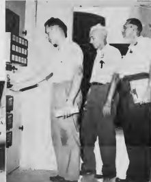
WHEN THE facilities of the substation had been checked out, the air circuit breaker on a Lago feeder was moved from its testing to operating position. OTRA CU e facilidadnan di e substation a worde checke, e interruptor di aire ariba un cable di Lago a worde movi for di su posicion di test pa posicion di operacion.
